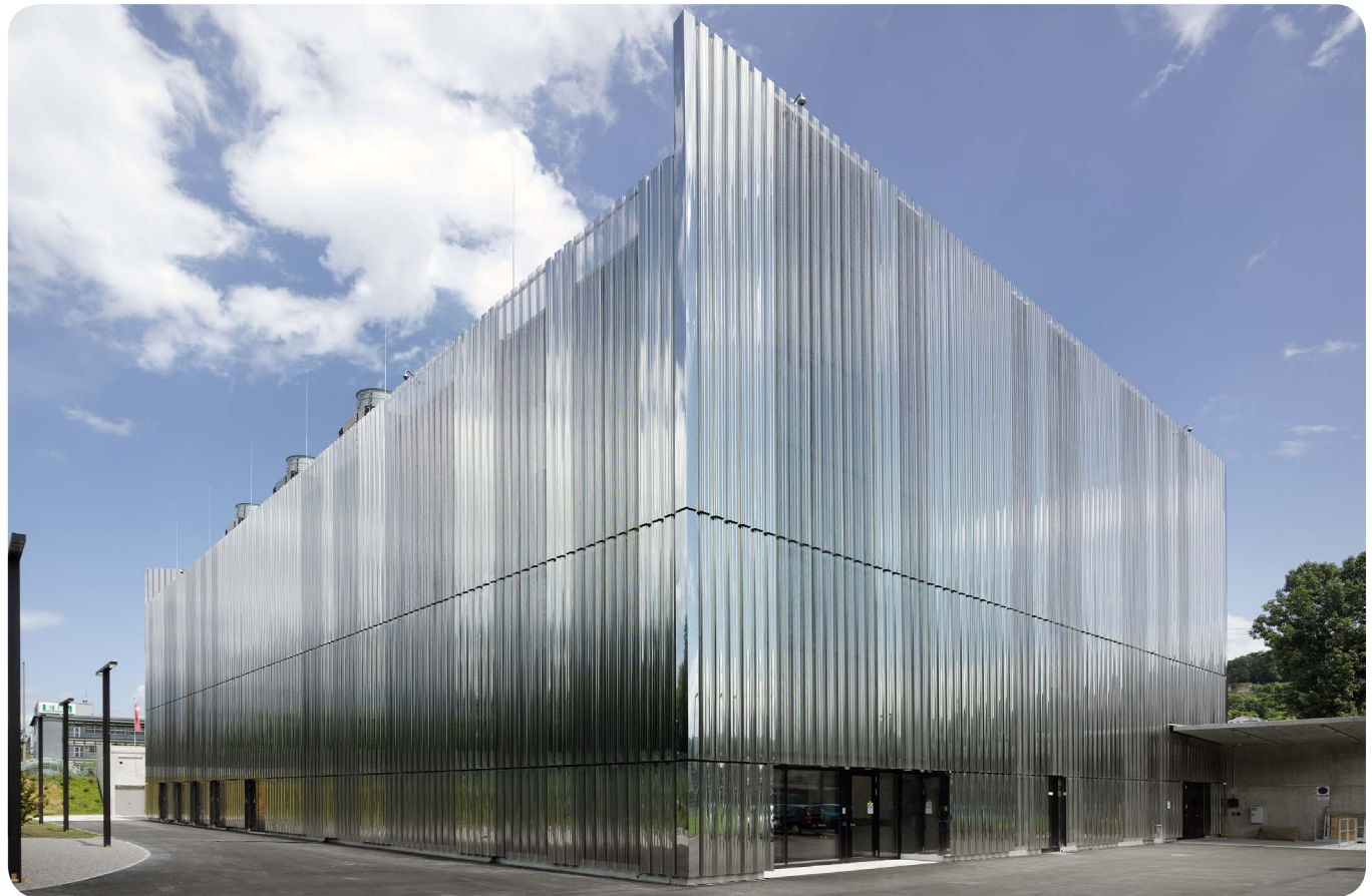
Picture courtesy of © Johannes Marburg Photography Geneva, Switzerland
